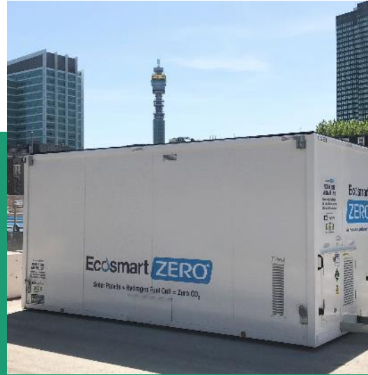
Stationary power for welfare cabins on HS2 sites
