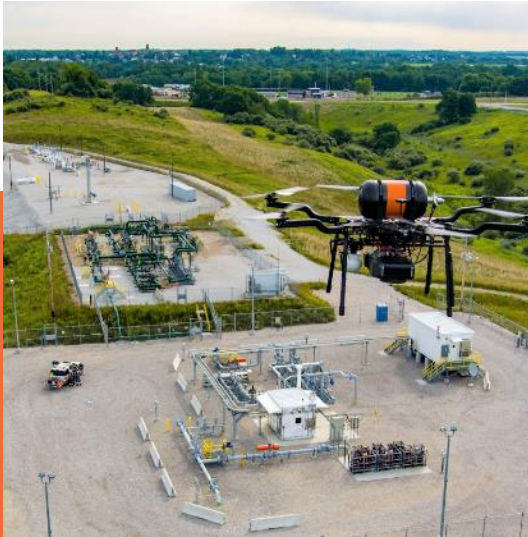
Pipeline inspection with Shell
