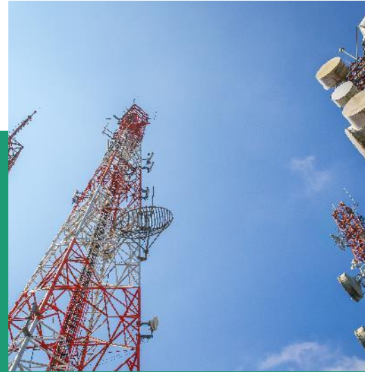
Back up power systems for telecoms sites with Netis
