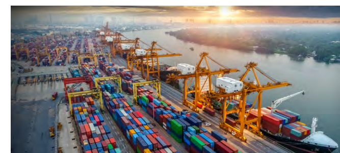
PORTS - SHORE-TO-SHIP POWER
